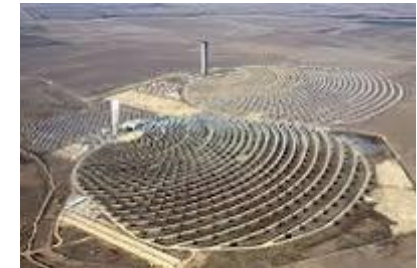
PS20. Power tower
