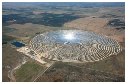
Gemasolar plant. Power tower
