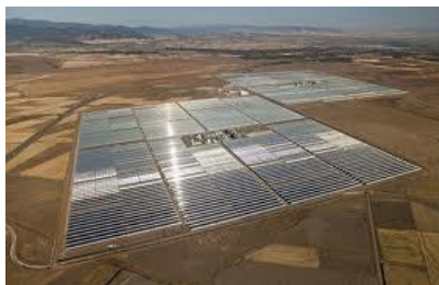
Andasol 1 and 2. Parabolic troughs
