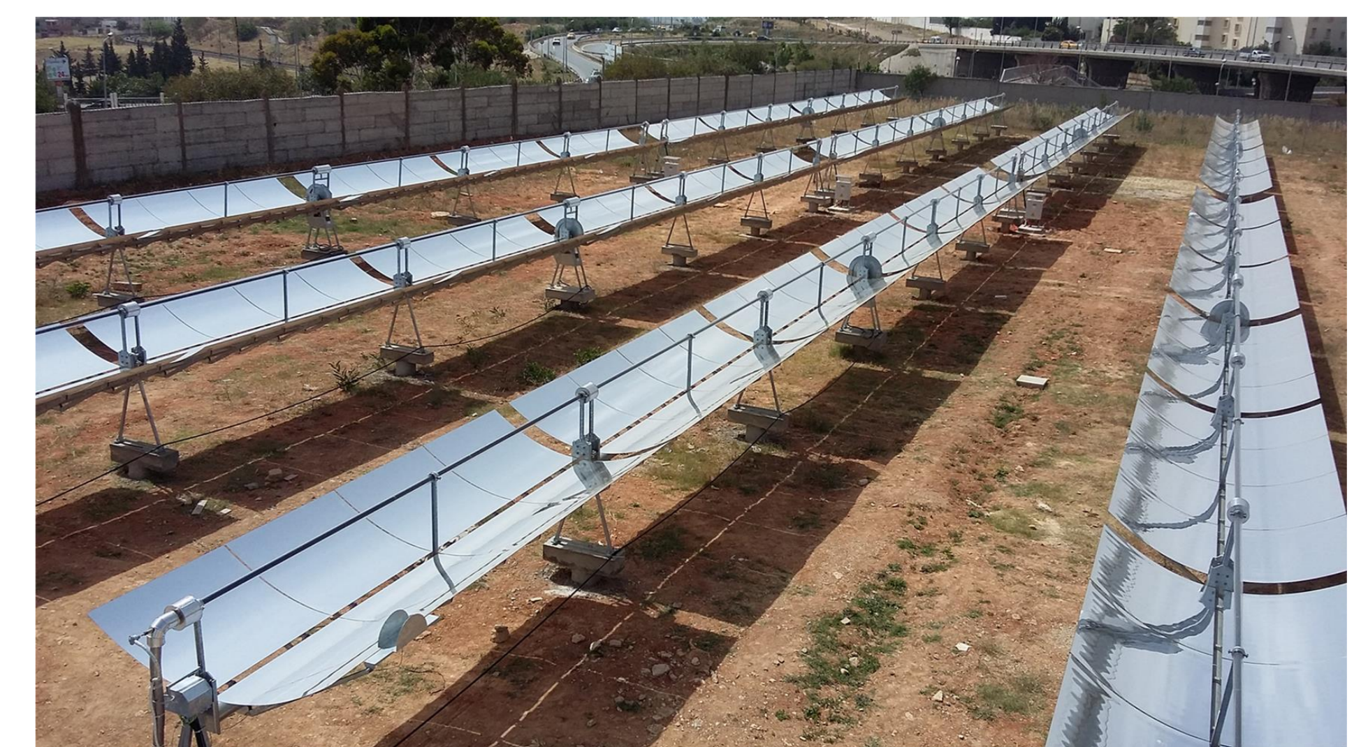
Figure 1. REELCOOP CSP/Biomass power plant prototype design (top) and parabolic through solar field installed in ENIT, Tunis (down).
