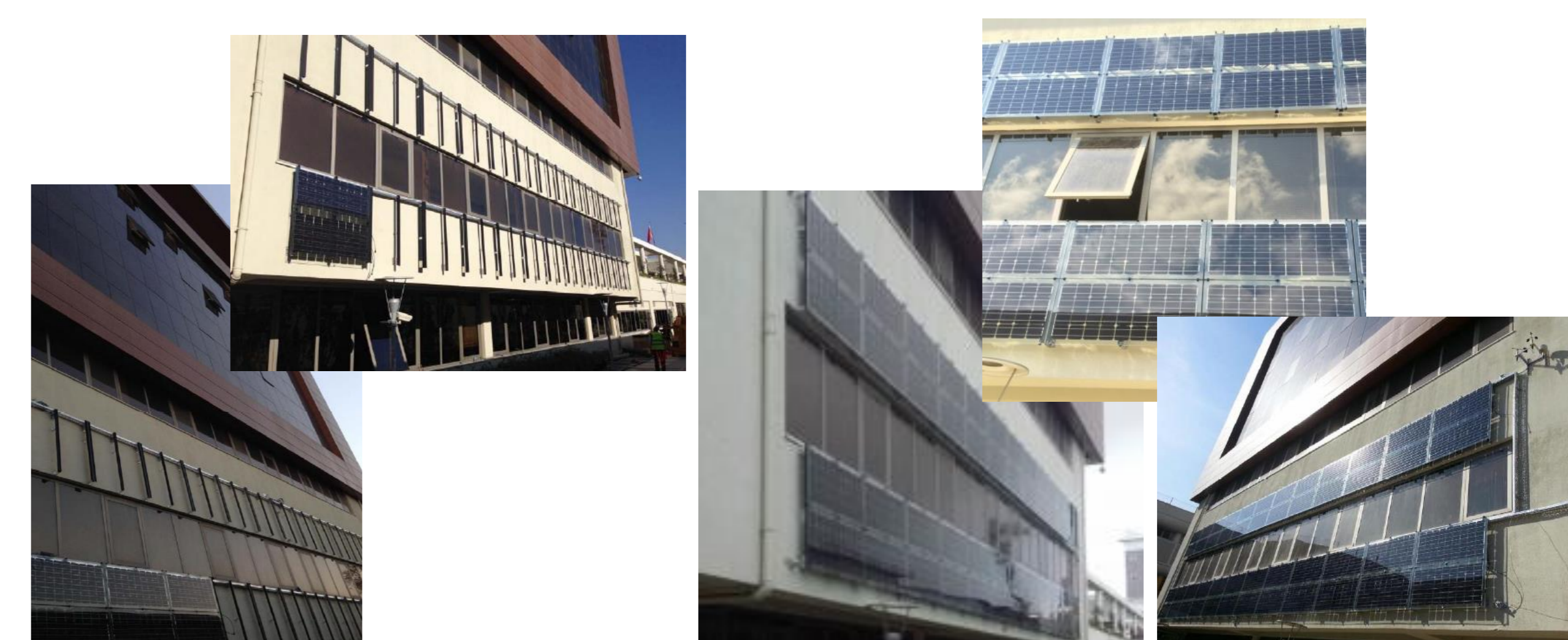
Figure 2. PV modules installation process at Yazar University, Izmir.
